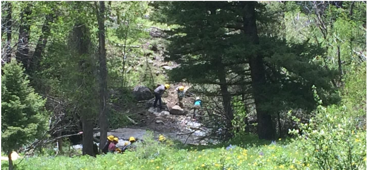
SCA crew constructing stairs on each side of Williams Creek.
