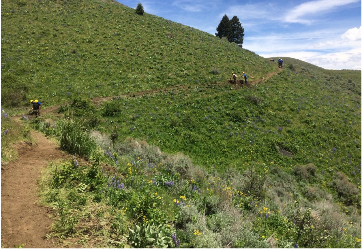
SCA crew armoring and retreading the Williams Creek Trail
