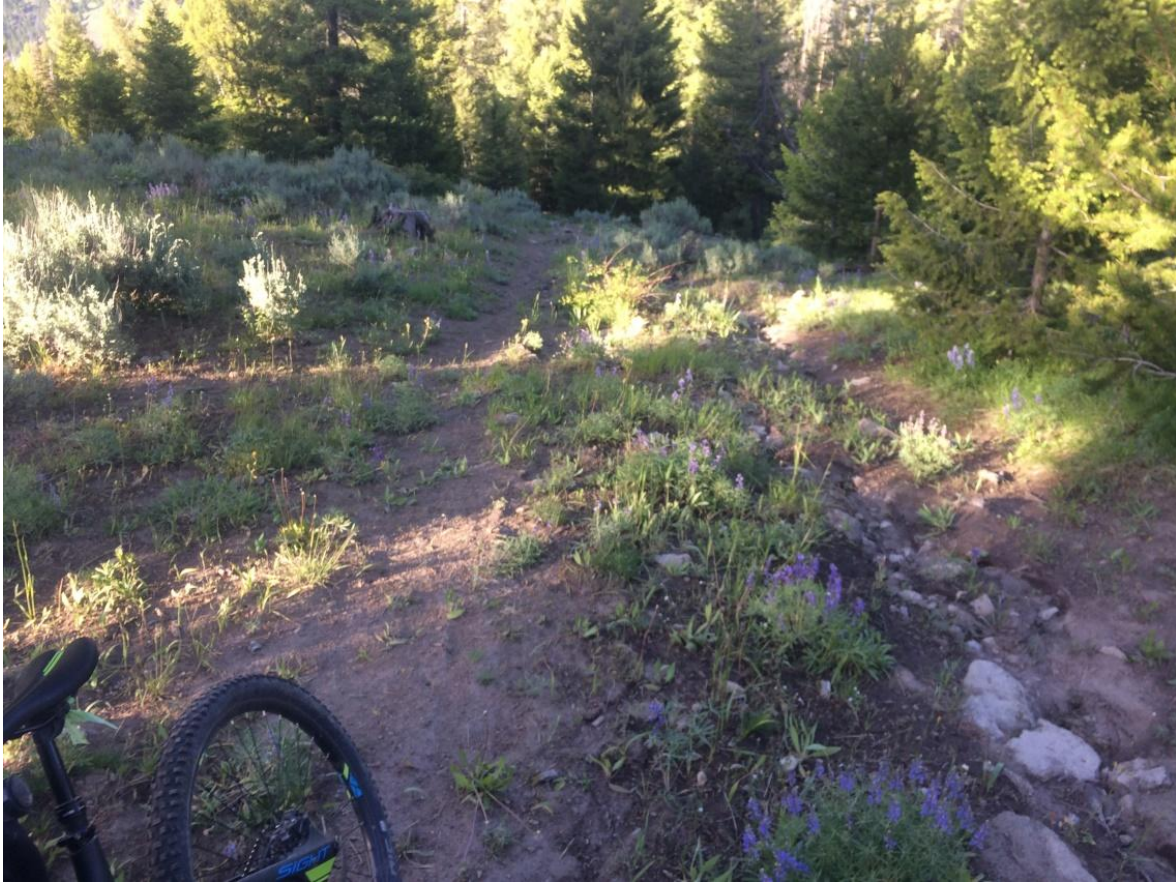
12 Mile Meadows Trail (101) is a fall line trail that has multiple braidings due to erosion.
