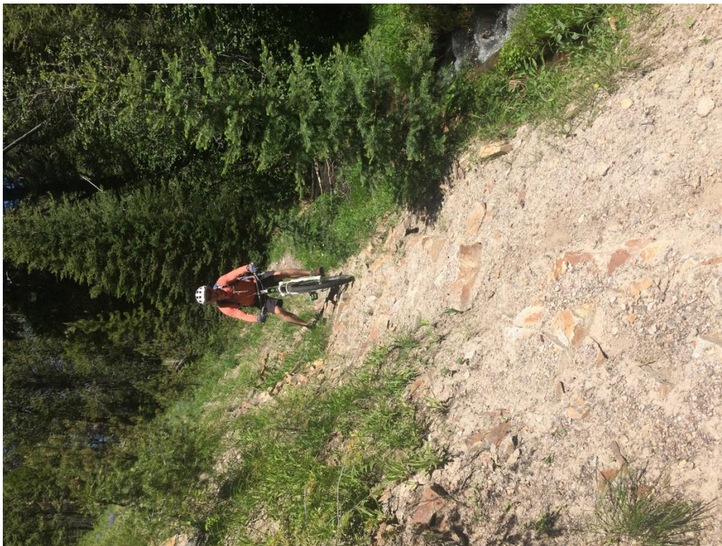
There are a few sections that need to be rebuilt.
