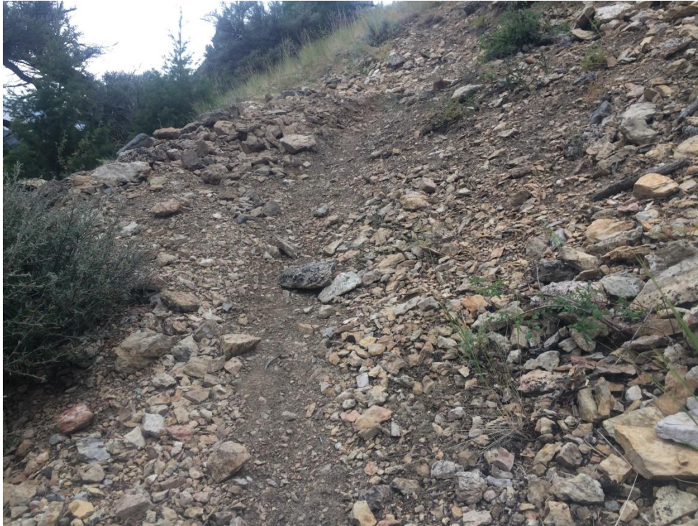
The Lime Creek Switchbacks. These were taken a month after the volunteer trail day. These are the ruts that were created when dirt bikers tried to make the tight turns. We need signs to inform them which trails are motorized and none motorized.
