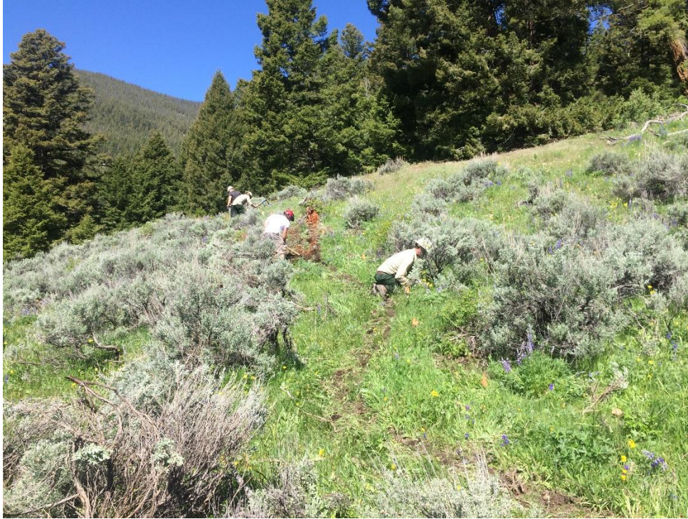
Clearing Vegetation and digging tread.
