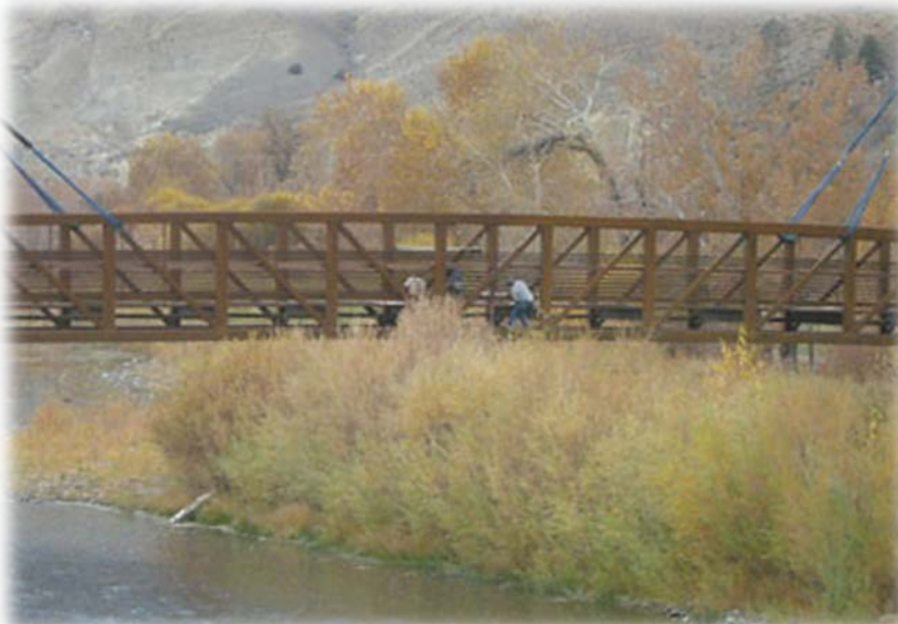
Pedestrian Bridge at Island Park
